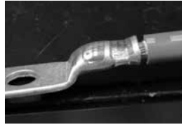
8. Completed crimp. Readjust the guide plate for the second crimp.
